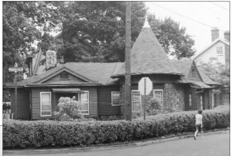
One of the two Gatehouses at Watsessing and Berkeley Avenues. Photo 1974
